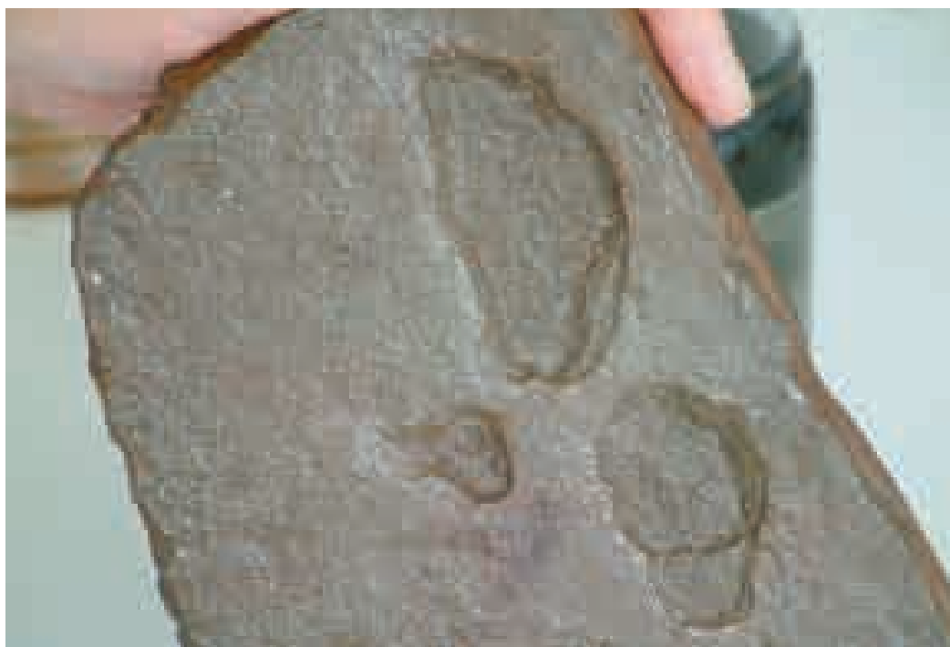
Tank bottom plate showing pitting corrosion by SRB
